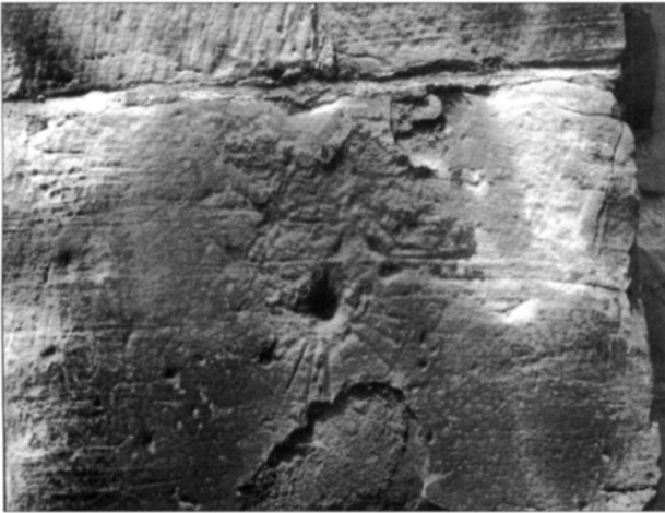
Fig. 2 Scratch Dial on buttress
